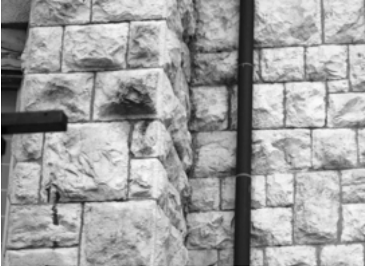
Figure 5: Wall Detail. Andrásy út, Budapest. Author's own (30 Dec 2014).
