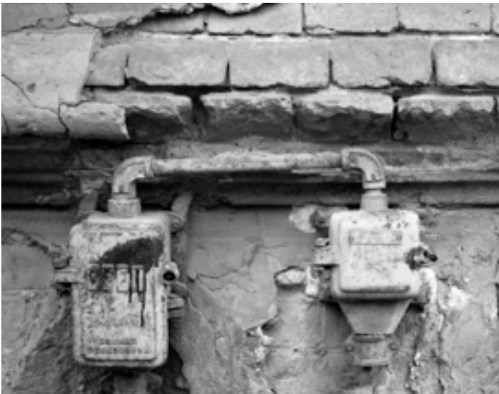
Figure 6: Wall Detail. Andrásy út, Budapest. Author's own (30 Dec 2014).
